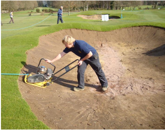
LEFT: Wacker plating bunker base: Similar practice used for adding new sand RIGHT: Good example of major ditch work and trimming back vegetation
